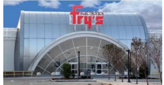
Fry's Electronics, 148,000 square feet of state-of-the-art electronics, choose Webster for its Space Station-themed electronics destination.
