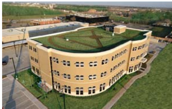
251 Medical Center Boulevard's living roof, the largest in Texas, is just one of the features in this innovative facility.
